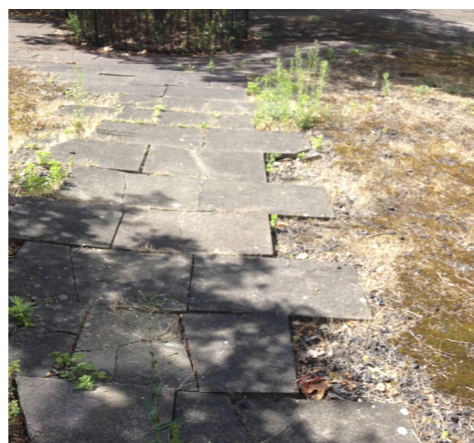
AREA A = The triangle is a passers by area. The existing pavement is in terrible condition with broken slabs and cracked tarmac throughout. The area is used by gangs at night as a space for dealing drugs.
