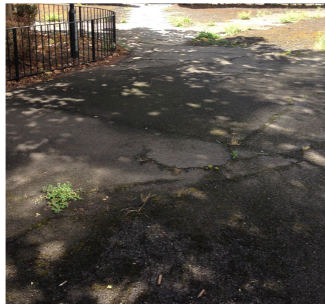
AREA A = The triangle is a passers by area. The existing pavement is in terrible condition with broken slabs and cracked tarmac throughout. The area is used by gangs at night as a space for dealing drugs.
